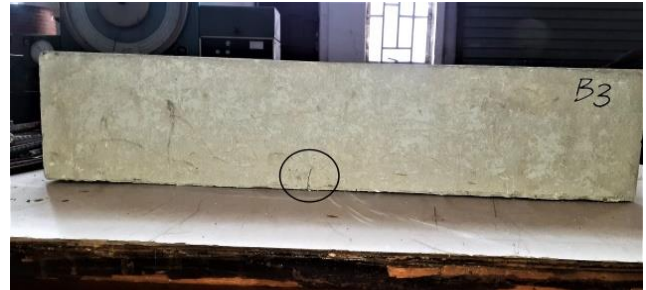
Figure 3: Picture showing first crack on the hollow cored beams that emanated due to the point load on a Type 2 Beam
