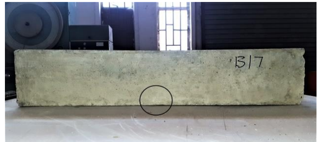
Figure 2: Picture showing first crack on the hollow cored beams that emanated due to the point load on a Type 1 Beam
