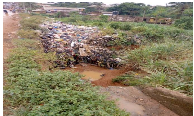
Figure 10: Itele road Dump site
