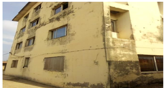
Figure 1: Typical assessed building
