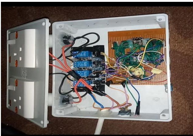
Figure 4: Components connection before closure
