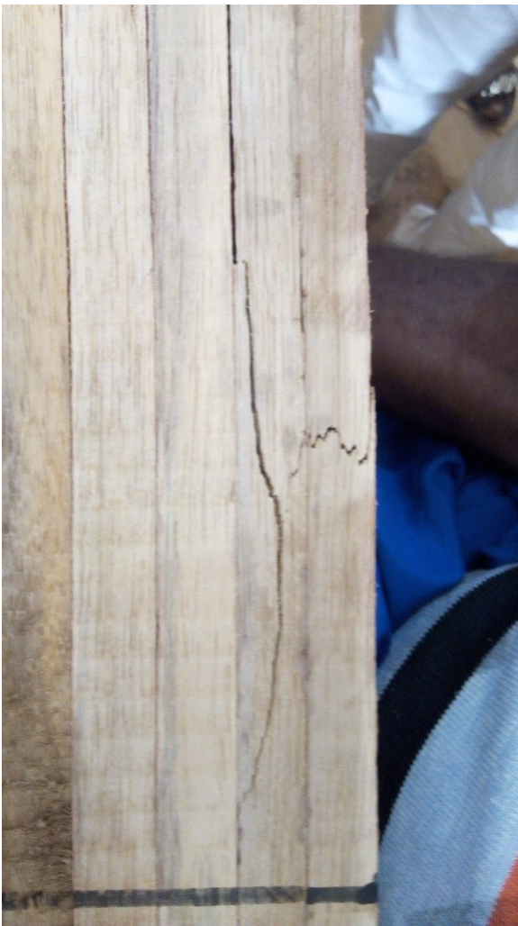
Figure 5: Section through the beam showing failure.
