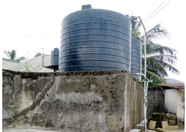
Figure 1: An elevated concrete water stanchion.
