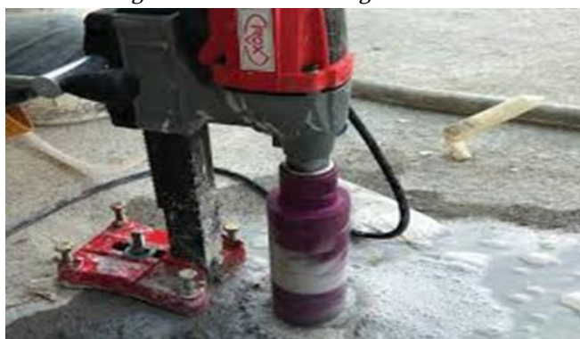
Figure 3: Floor Coring Operation Ongoing
