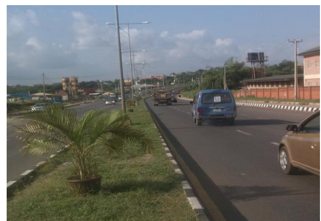
Plate 2: Improved Highway along Abiola way in Abeokuta City. Source: Author Field Survey, 2017.
