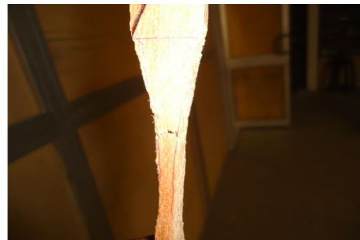
(b) Failure mode showing crack
