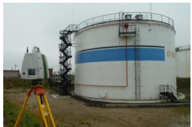
Figure 2: TLS and Reservoir
