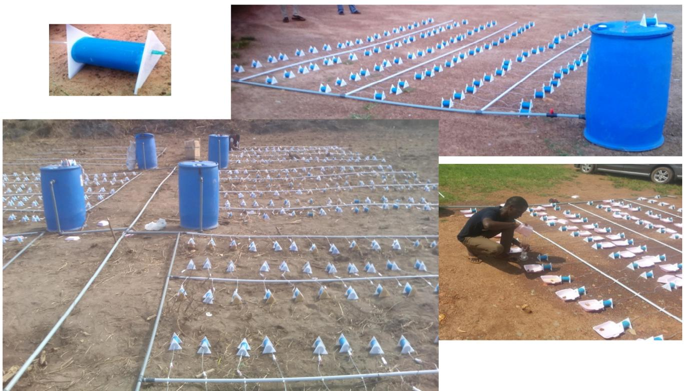
Figure 3: Installation of low cost drip system on the field and discharge measurement
