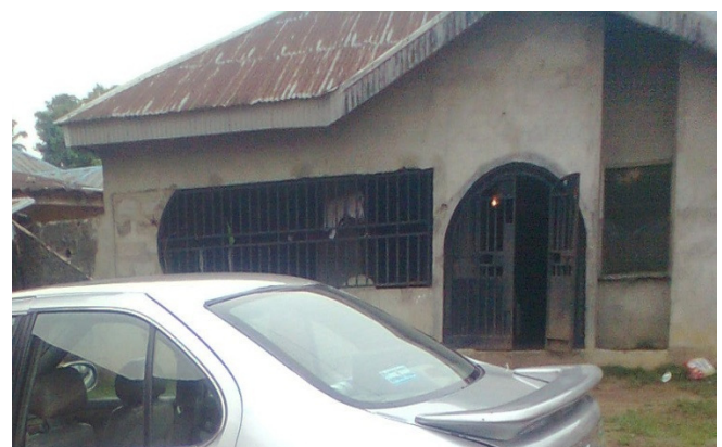
Figure 6: Sandcrete Building with Rusted Corrugated Iron Sheet Roof
