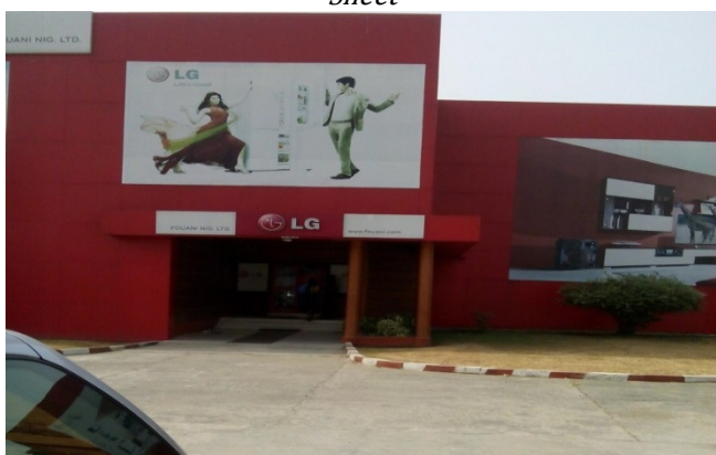
Figure 5: Building with Alucoboard Wall Cladding
