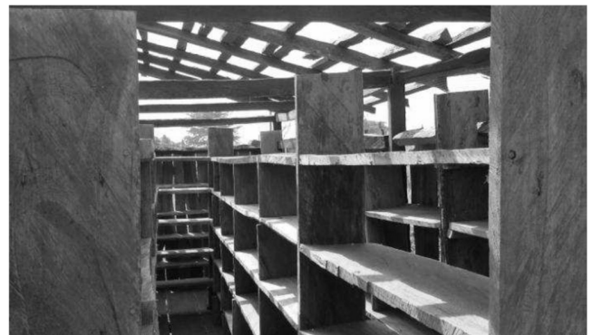
Figure-1: Yam Storage Chamber Constructed with Ceiba Wood
