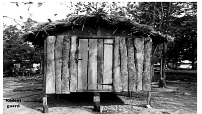
Figure-2: Complete Yam Storage Chamber with Rodent Guards Fixed
