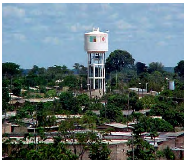
Figure 8. One of the tanks used to distribute water in George compound.
