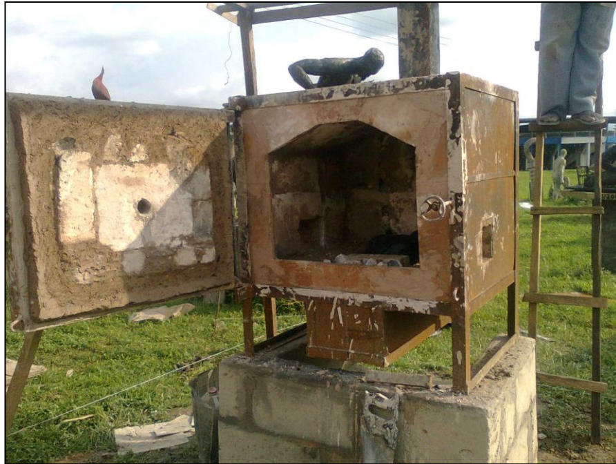
Plate 6. The Kiln near Completion.
