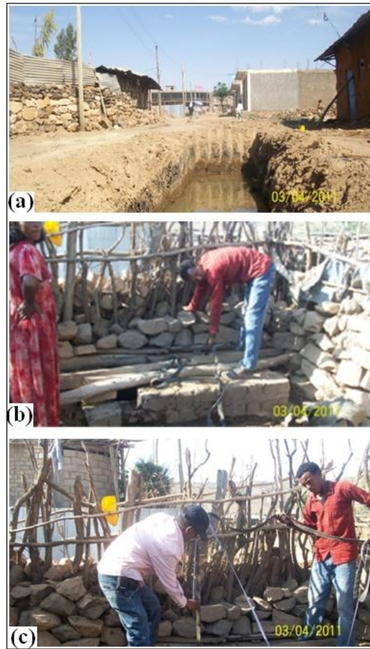
Figure 8. Shallow groundwater in (a) trench excavated for drainage line installation (b) and (c) groundwater level measurement from house hold hand dug wells.
