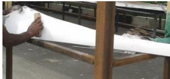
Figure 15. Filling the holes and smoothing the wind turbine blade.
