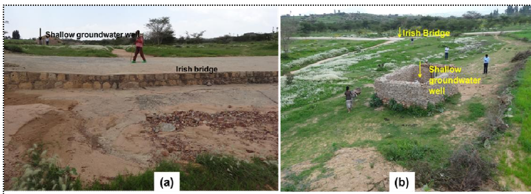
Plate 7. A shallow groundwater well (for water supply) developed at upstream of an Irish bridge in northern Ethiopia (a) Upstream view and (b) downstream view.
