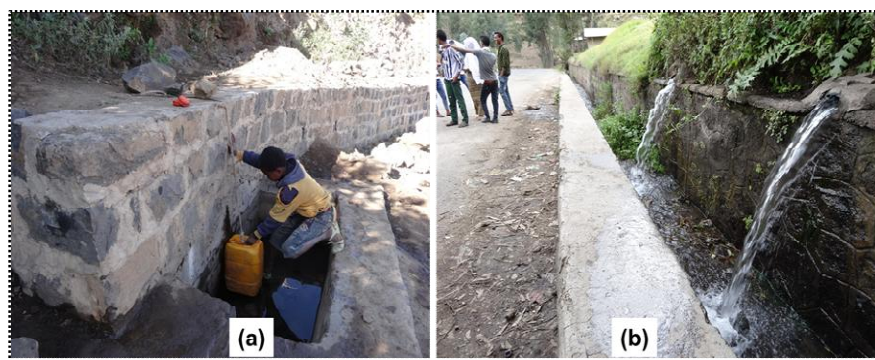
Plate 11. Spring developed from a road cut in northern Ethiopia: (a) for rural water supply, and (b) for small-scale irrigation purpose.
