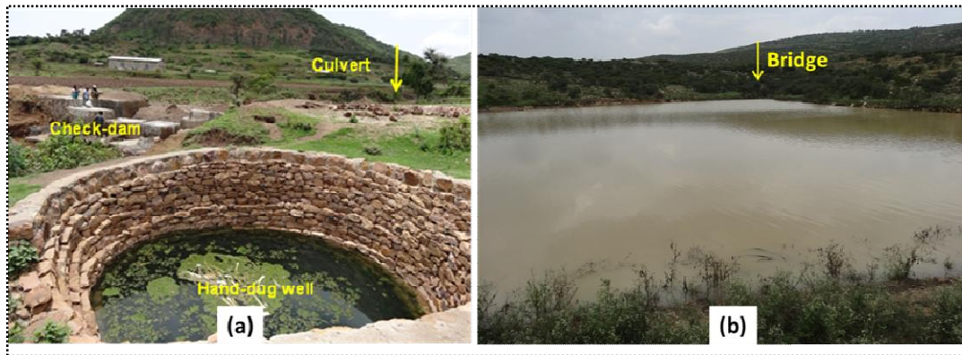
Plate 5. Water from road catchments is channeled into water storage structures for surface water harvesting and groundwater recharge in northern Ethiopia: (a) water from a culvert is stored in a check-dam pond, and (b) small dam is used to store water from a bridge.
