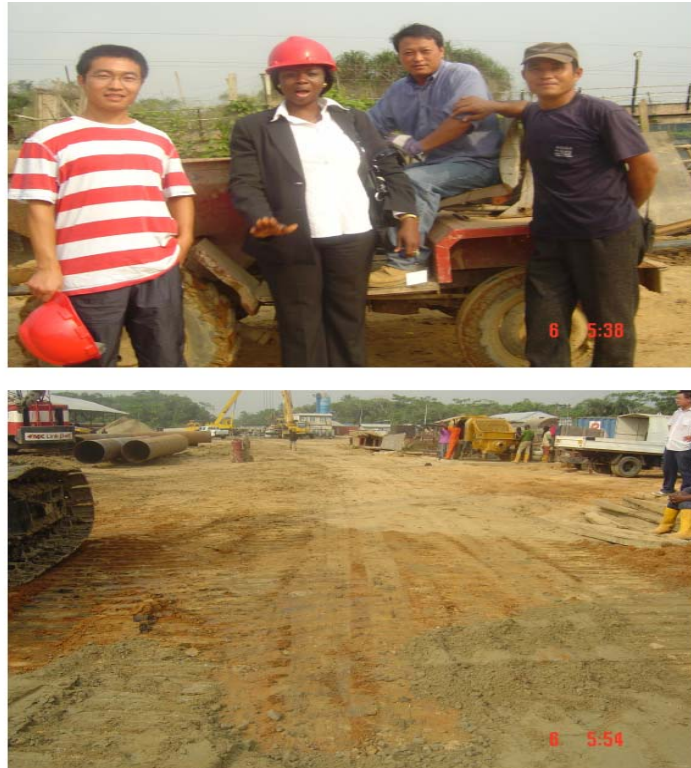
Figure 1: The author (center) with Chinese construction workers (above) and the road under construction at Idundu, near Calabar (below).
