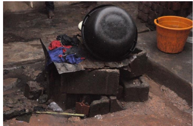
Figure 12: Uncovered dumped well
