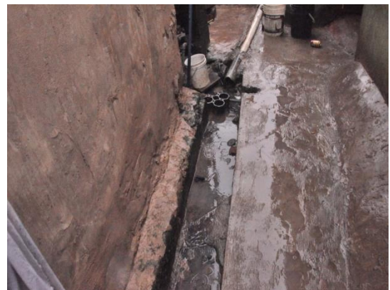
Figure 20: Open drainage system in the area
