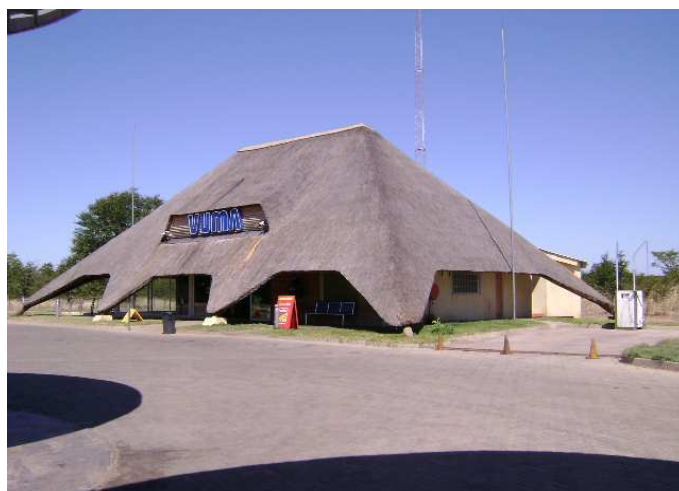
Fig. 3: A fuel filling station in Livingstone, Zambia roofed with thatch (Source: Authors')
