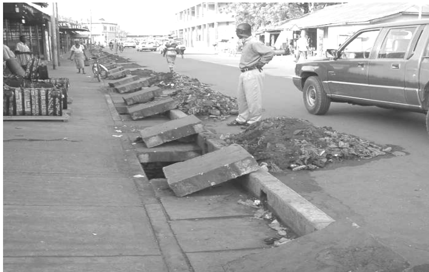
Plate 1: A silted covered roadside concrete U-drain in Tamale being desilted
