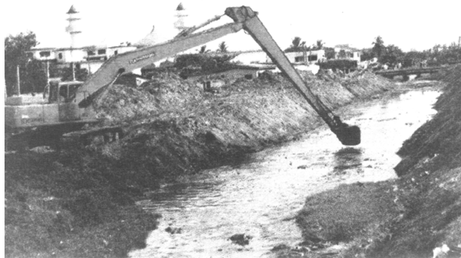
Plate 2: Desilting of a Stream Channel in Accra
