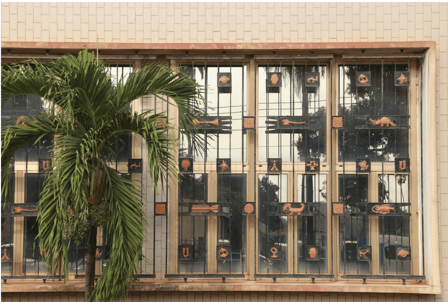
Figure 11: Details of ornamentation on the front façade of BoG Office, Kumasi showing the goldweight symbols casted in metal and finished in bronze colour (Photo source: Author)
