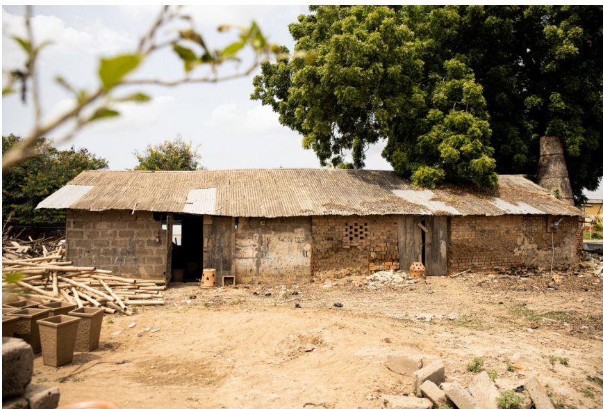
Figure 4: The structure built by Michael Cardew in Vume for Women to practice pottery
