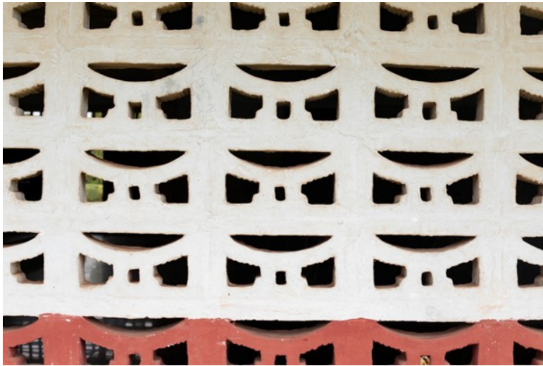
Fig. 1: Stool symbol cast in concrete moulding used as sunbreaks and ventilation device that is also appreciated for its socio-political and educational significance
