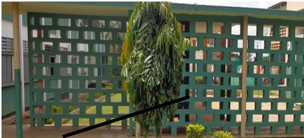
Fig. 5: The crocodile motif employed as simple geometric patterns in tessellating forms to create sunbreaks and lattices for the pathway that link the administration to other parts of Prempeh Senior High School
