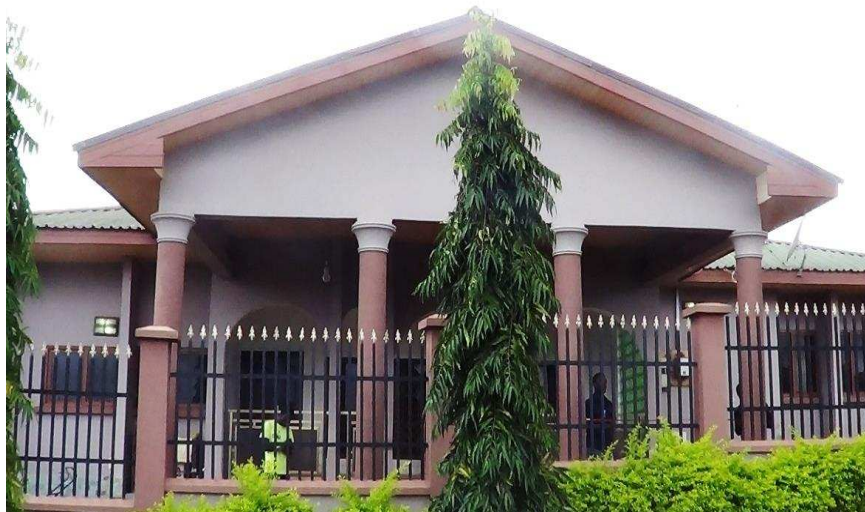
Fig. 4: Front part of the building under study
