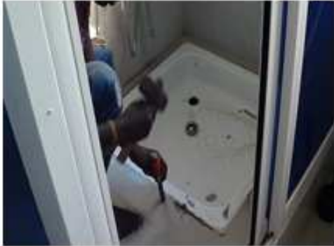
Fig. 18: Shower tray being removed to check the situation underneath
