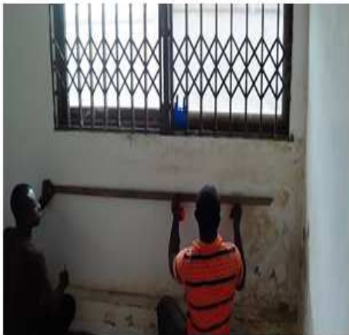
Fig. 2: Marking grid points with light wooden batten
