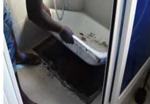
Fig. 18: Shower tray being removed to check the situation underneath
