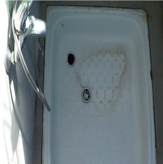
Fig. 17: Shower tray fixed in bathroom 1
