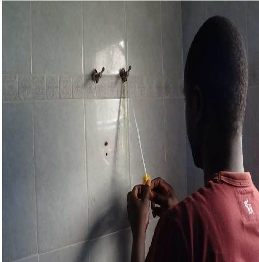
Fig. 16: Inspection of stop valves by a plumber
