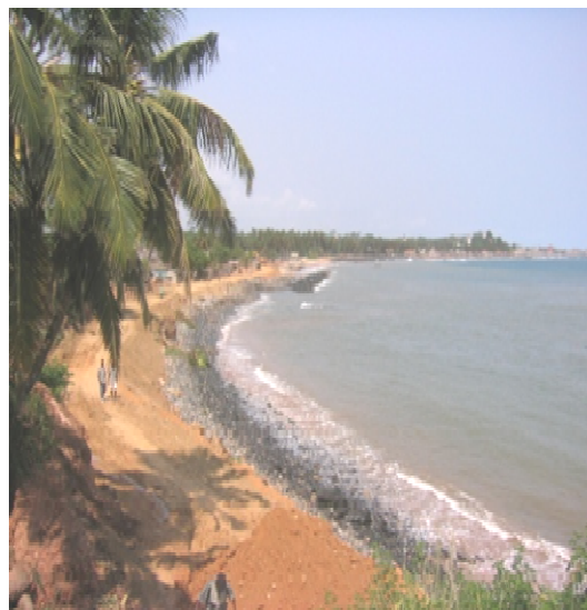
Plate 2b: An eroded street of the community is being reconstructed
