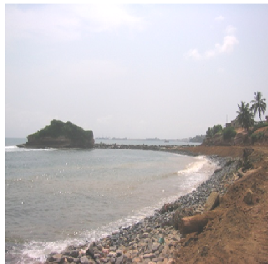
Plate 4: View of the Shoreline of Nkontompo showing the protruding end detached from the mainland (Source: Photograph from authors' field survey, Nov. 2003)
