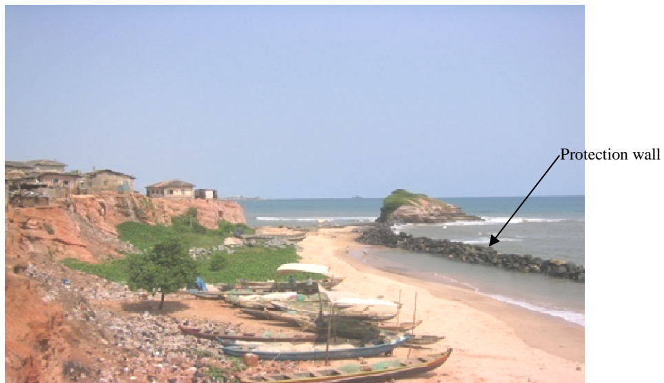
Plate 1: Shoreline has receded beyond the protection wall in place
