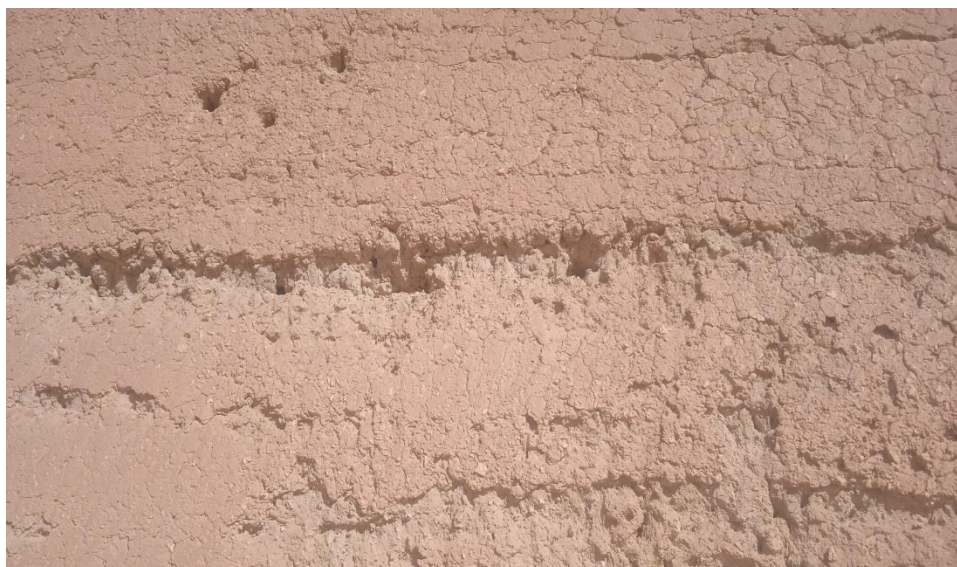
figure 04: The image illustrates the impact of wind on the northern wall of Kasr Melouka Source: The researcher.
