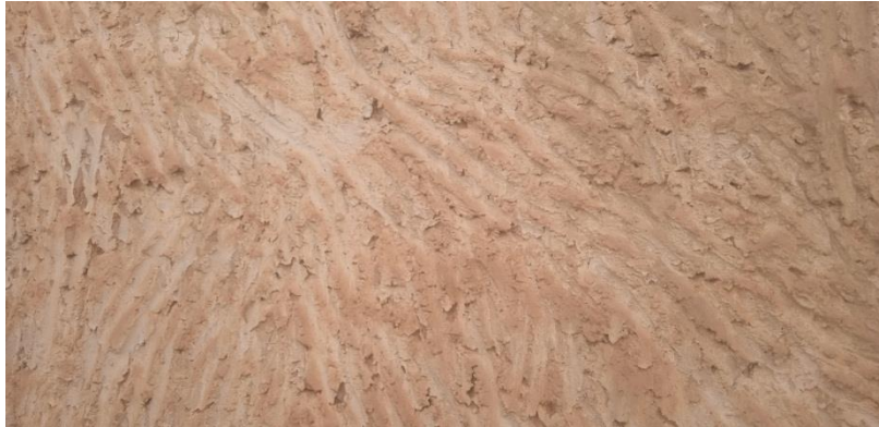
figure 01: The image illustrates the use of hands in plastering the walls.
