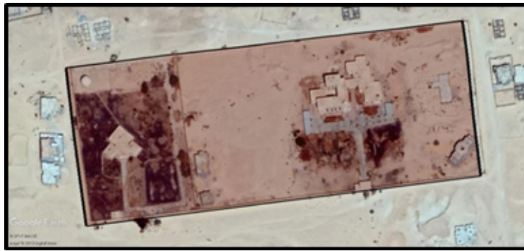
Fig. 3. Aerial view of the Libyan Center for Desert Research and Desert Community Development.
