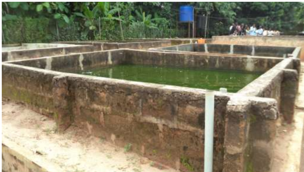
Plate 6: Pond F (Surface concrete pond)
