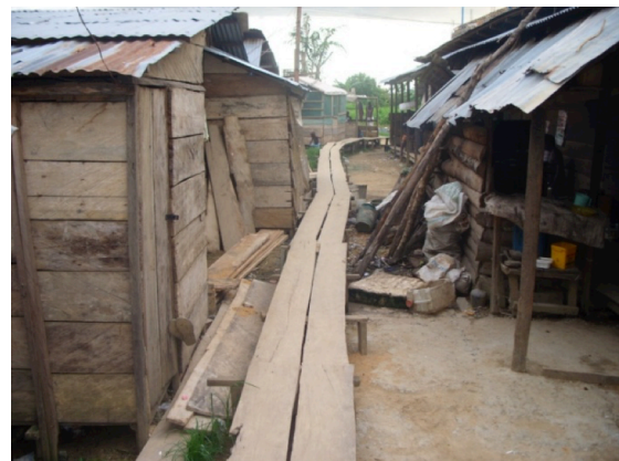
Fig 9 Raised walkway running the entire length of the IDP camp
