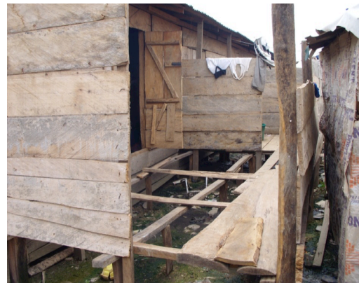
Fig 6 Showing bathing space behind the building
