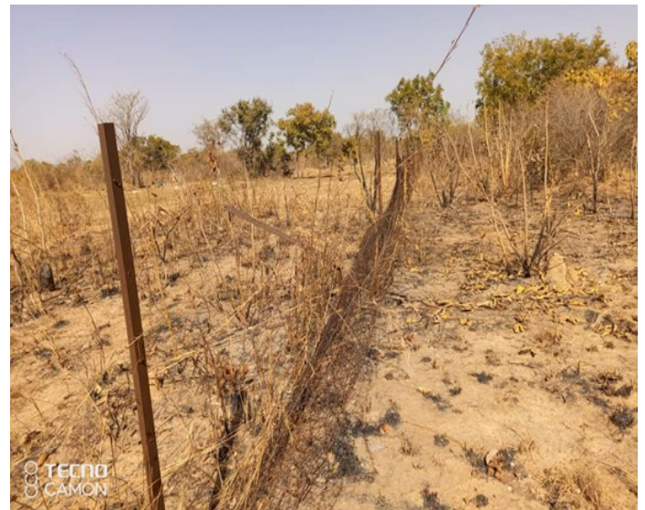
Figure 8 Portions of broken wire mesh fencing
