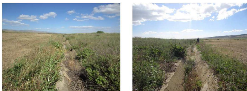
Fig.8. Images of the drainage channel
