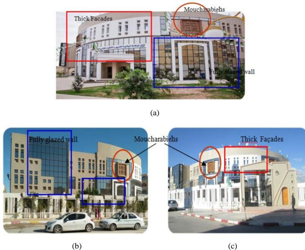
Fig.3. The case study building.
