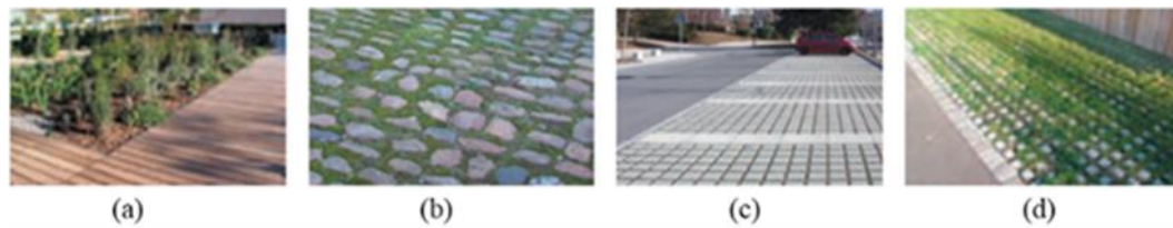
Fig.8. Different types of permeable covering floor and their uses. (a): Plate of wood, (b): Natural stone pavers, (c): Concrete pavers, (d): alveoli slabs [9]
