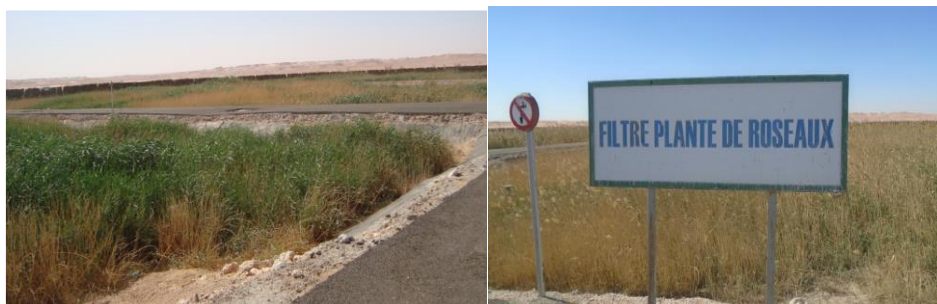
Fig.4. Reed Plant Filter
