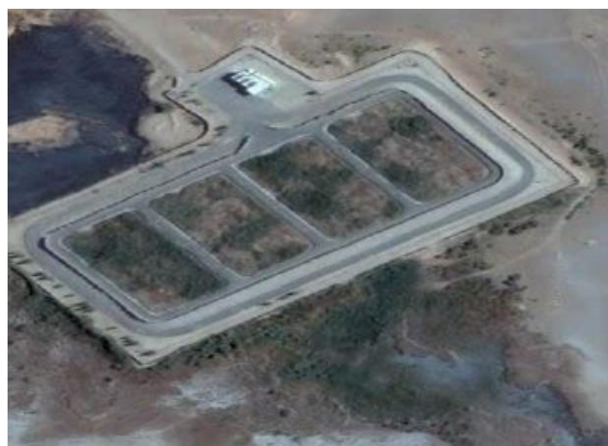
Fig.2. Wastewater Treatment Plant N'GOUSSA
