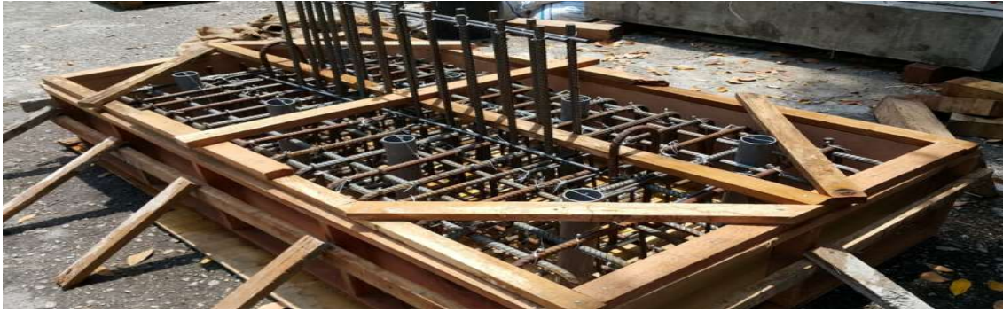
Fig.2. Preparation of foundation beam cage
