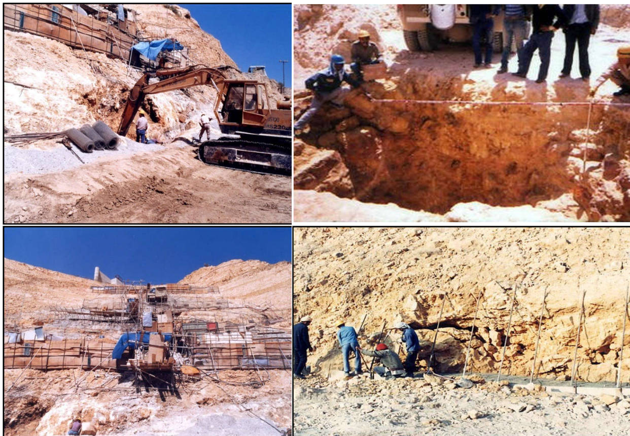
Fig.6. Geological survey (source: ANDT 2010).
