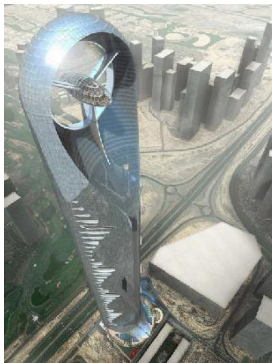
Fig.12. Overview of the Tower
