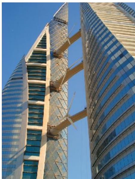
Fig.5. A view of locating three wind turbines between two tower buildings
