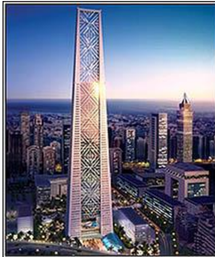
Fig.9. Overview of the Tower
