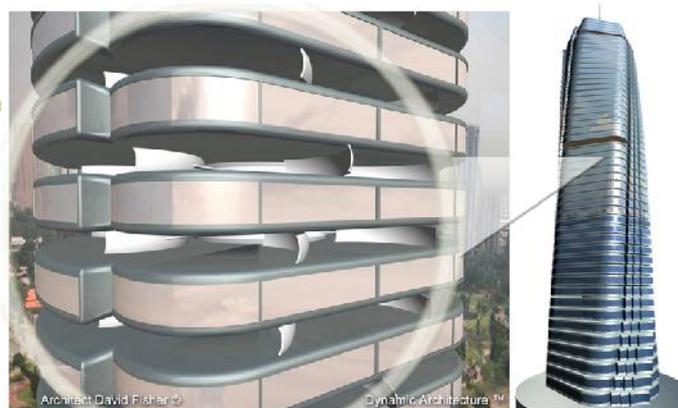
**Fig.7.** the turbine location between floors
