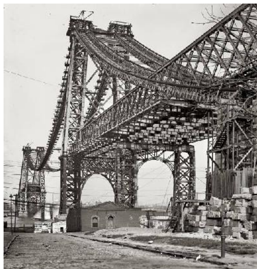
Fig.5. Williamsburg Bridge, 1924. In 1988 the poor condition of the bridge became an emergency [28]
