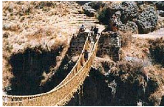
Fig.8. Traditional local rope structures: Inca's suspension bridges [36]
