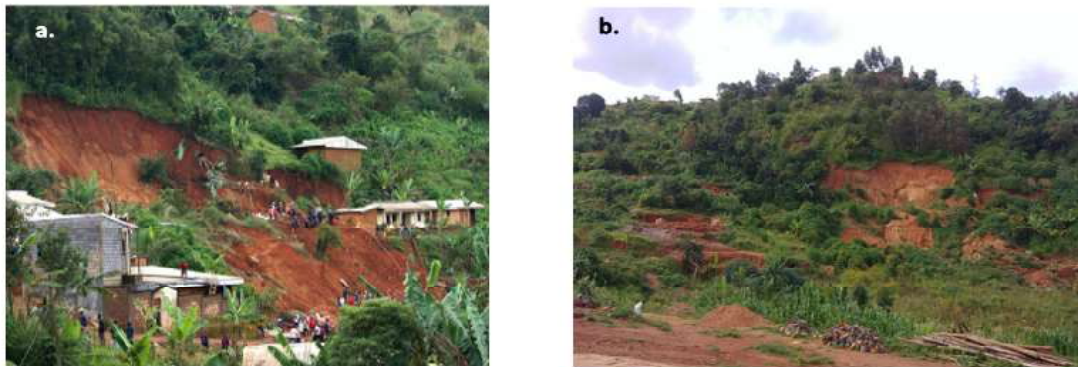
Figure 8: Landslide site at Gouache showing: a) the landslide scar in the centre and buildings that were unaffected at the side of the scar; and b) demolition of these buildings after the landslide event
