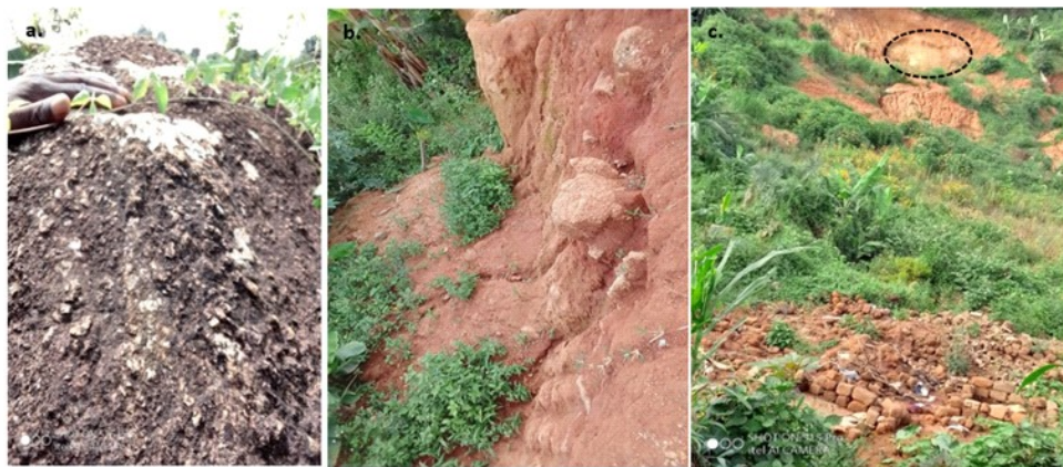
Figure 4. Geology of Gouache at the landslide site showing: a) Fresh granitic rock, b) clayey soil with intercalations of weathered granites and c) landslide scar
