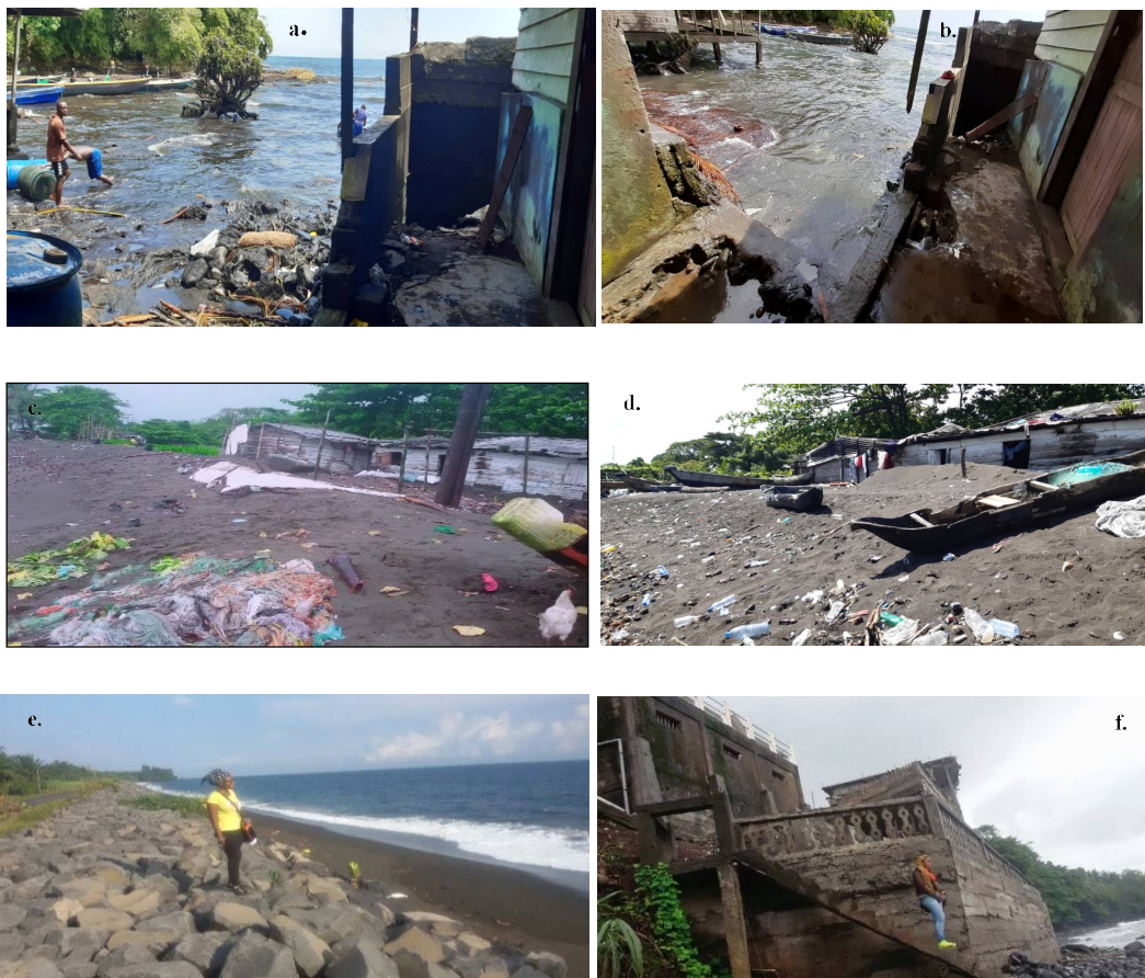
Fig. 9: Coastal protection measures implemented at the West Coast showing a & b. embankments at DFP, c & d. use of sand bags at DFP, e. rock embankment protecting the highway at the West Coast and f. seawall (embankment) at Batoke.
