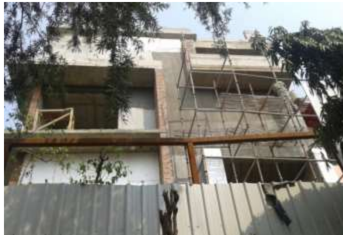
Fig. 16. The insulated EPS tiles cladding on external walls.
