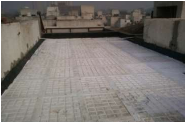
Fig. 14. The final finished roof surface with insulated EPS tiles.
