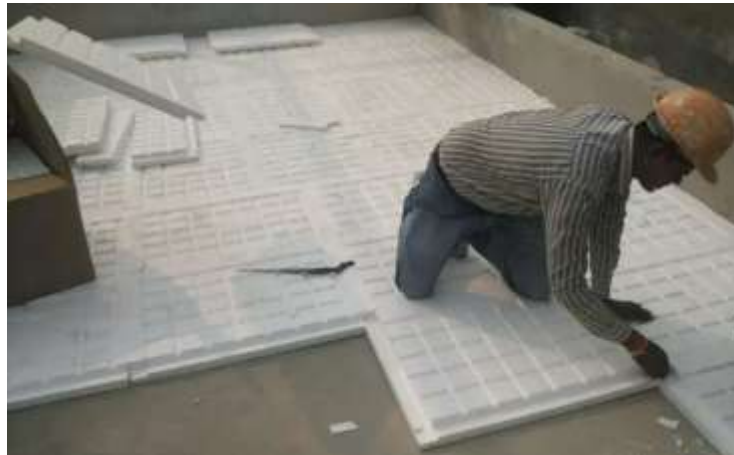
Fig. 13. The interlocking insulated EPS sheets laid on the terrace.
