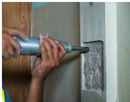
Fig.7: Schmidt Rebound Hammer
