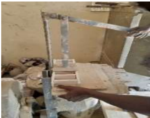
Plate 9: Manual Compaction of Clay-Brick
