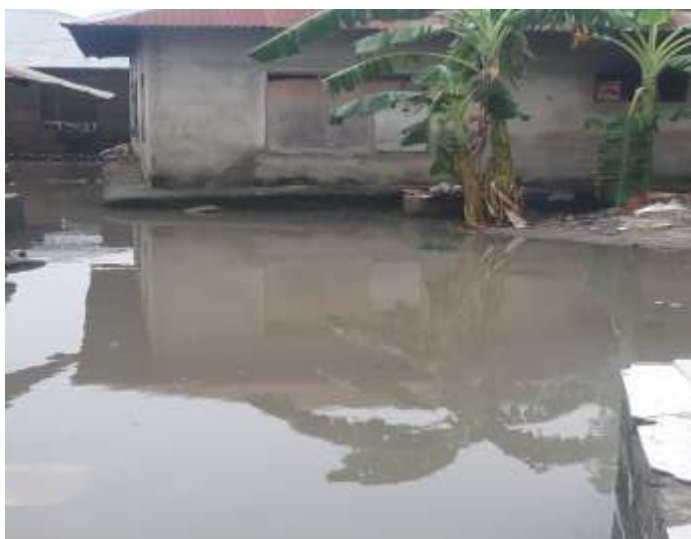
Fig. 1: Septic tank overflow due to rainwater entry
