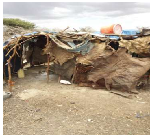
Fig 5: A photograph of a typical structure constructed with animals' skins is shown. Source: Field Survey, 2022
