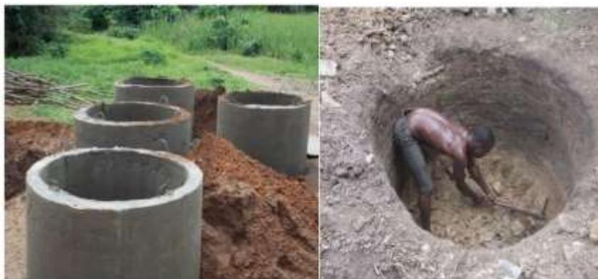
Plate 1: 1 m high concrete rings for lining the wells and excavation of a hand-dug well
