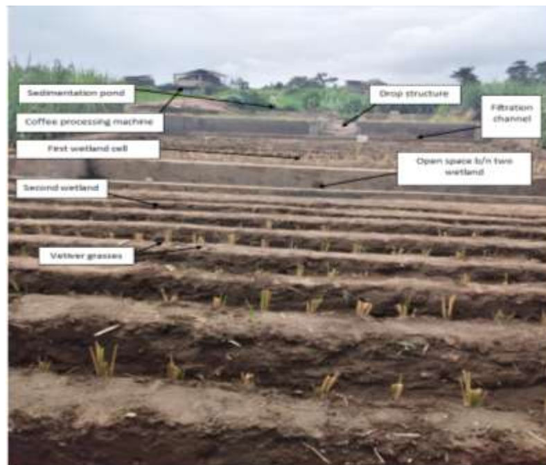
Fig 3: The whole system design of the constructed wetland
